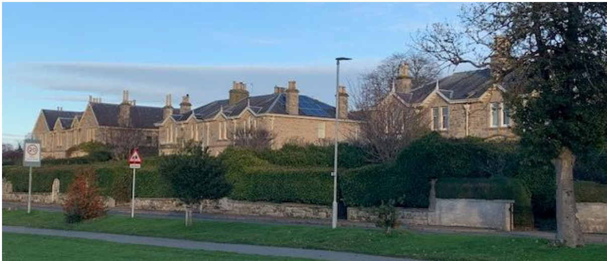
Figure 7: Stone Built Houses on Sanquhar Road
