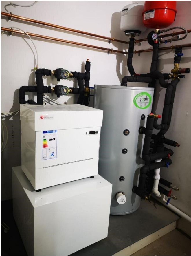
Figure 16: Kensa shoe box heat pump and small domestic hot water cylinder (e.g. for flats)
